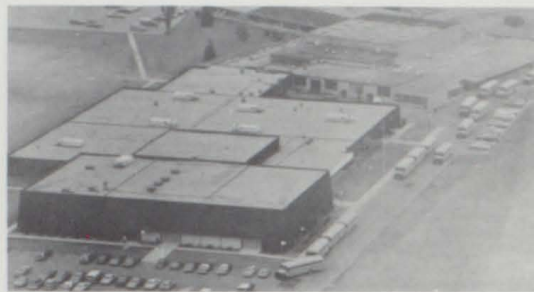
Aerial view of Seymour High School
