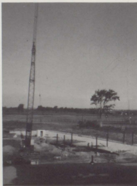
The foundations were laid.
