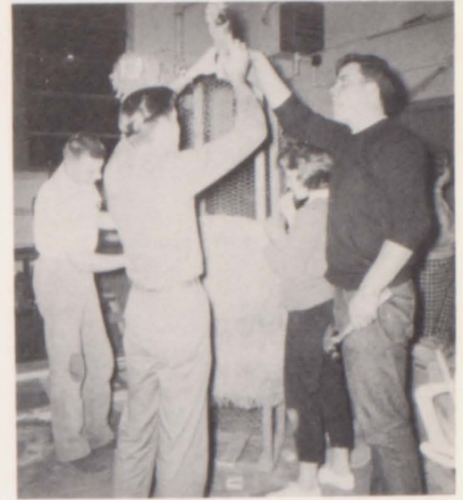
Ronald Dranzik, Chris Anschutz, Sharon Braun, Bill Maass, and Connie Husman construct the "Gopher."
