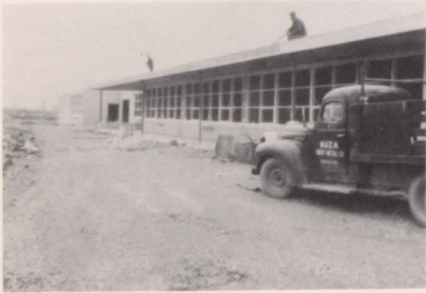
Late fall—the South Addition was well underway!
